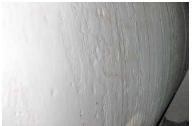
Tunnel Liner - 6 Months After Application
