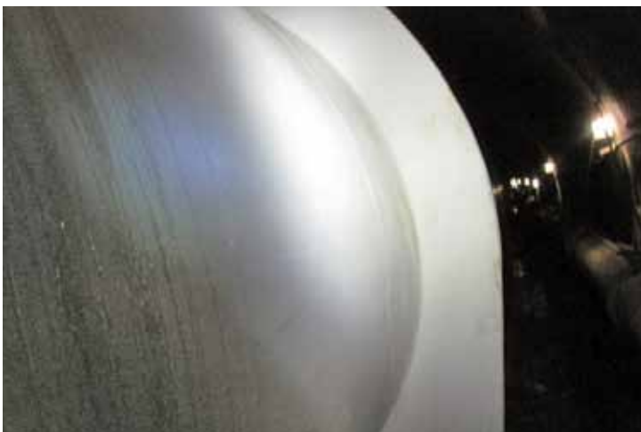
Tunnel Liner - 6 Months After Application
