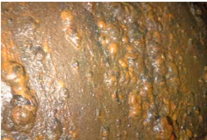
Tunnel Liner - Before Application
