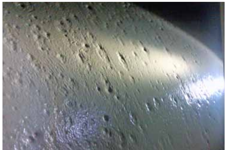
Tunnel Liner - After Application
