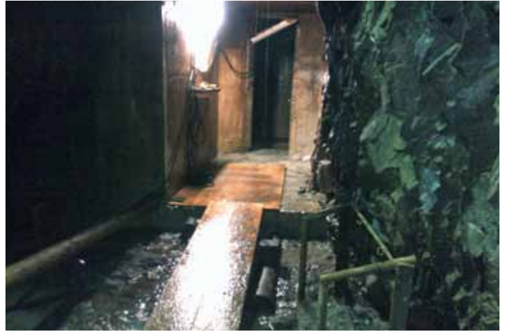
Entrance at the Bottom of Vertical Shaft
